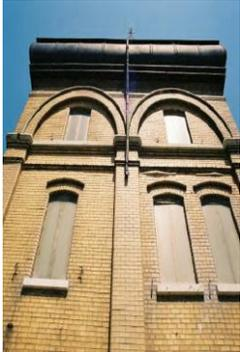
The first floor lighthouse windows are now concrete and the second and third floors are Plexiglas. These will all be replaced with strengthened glass and shutters.
